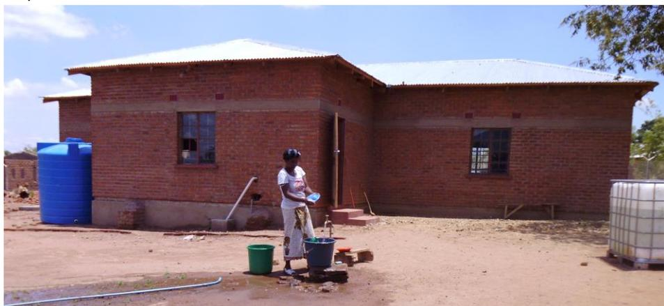
The bore hole is soon to be completed. Currently piped water is in use with a water storage tank with 5000 litres installed to act as stand by water storage.
